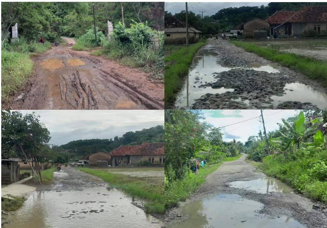
Figure 1. Visual documentation of the access routes to Cikadal Beach, highlighting significant accessibility challenges due to unpaved, potholed, and muddy road conditions. (source: author's documentation, 2025)
